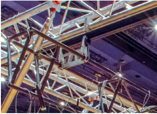
(a) The carbon truss is held in place by a roller bearing that can traverse along a rail.
