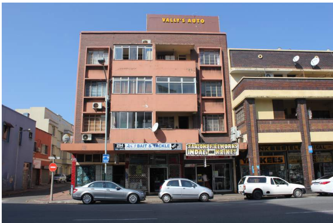
Figure 2: Afzal Building on 292 Grey Street.
